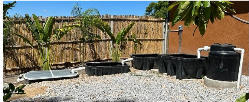
All stillage is treated by a multi-step system that includes de-acidification pools, an aerated algae pond, rhizome filtration system, and solar evaporator that returns clean, pH-neutral water to the local ecosystem.
